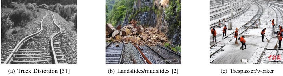
Fig. 13. Three types of railway anomalies. When a pilot vehicle detects trespassers or workers, it can ring the bell to warn and expel them, or brake itself (and its mother train) to protect them. Note that braking a pilot vehicle is much easier than braking its mother train, due to mass difference.
